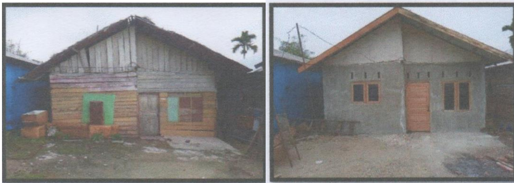
Figure 2. Renovation of Houses for the Poor
