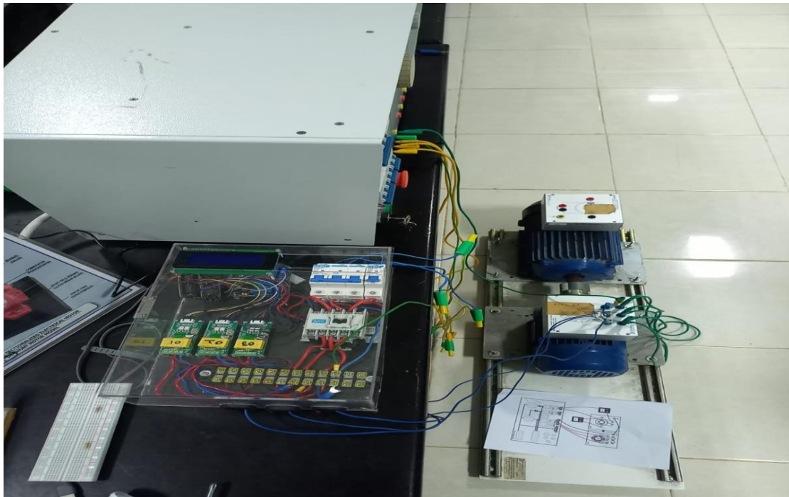
Figure 7 Realization of an IoT-based Three-phase Induction Motor Monitoring System
