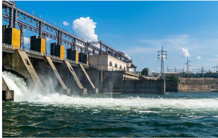
Figure 3. Hydroelectric power plant
