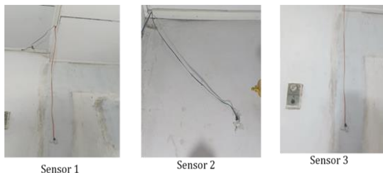
Figure 8. Room temperature sensor DHT22
