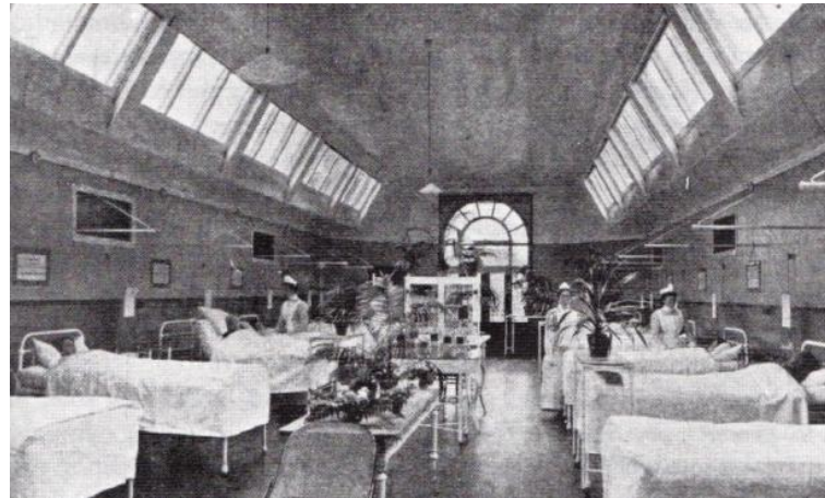
Figure 3. Ward interior Source: Adapted from [4]
