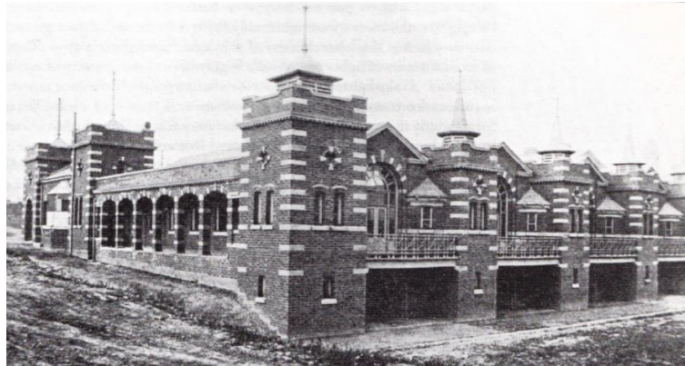
Figure 1. View of ward block from the South-East Source: Adapted from [4]
